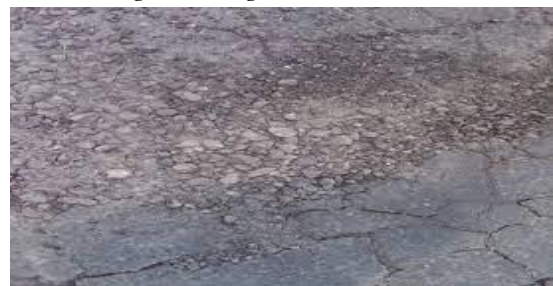
Gambar 19. Weathering/Raveling
