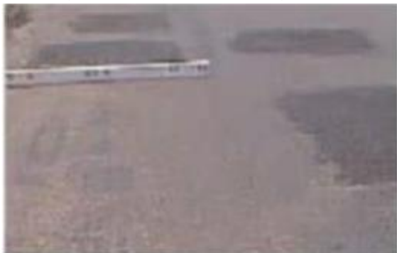
Gambar 11. Patching And Utility Cut Patching
